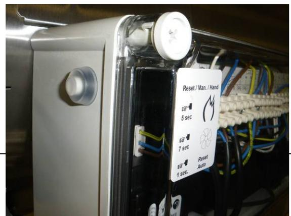
button is pushed again for 2 seconds the heater will stop. The heater will remain in the burn mode for maximal 24 hour. Every hour the heater will perform a safety shutdown and will automatically restart.
